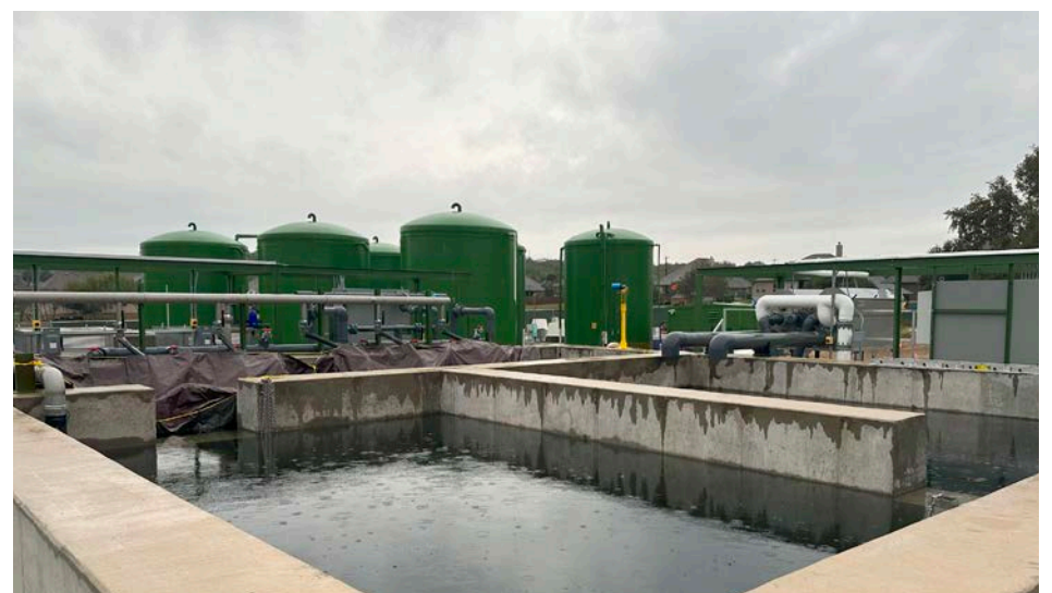
Photos above of the nearly-completed MBR plant.
